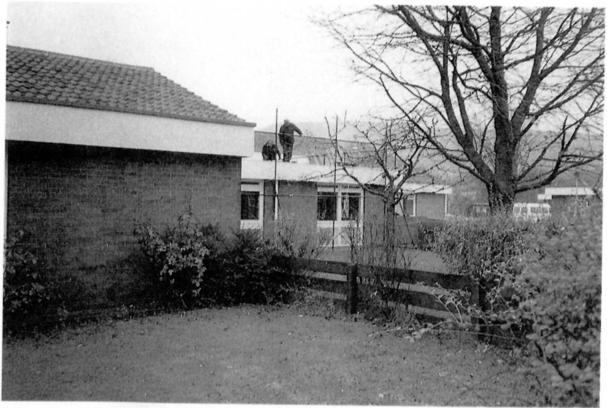
Rowley Jones Hostel under repair.
